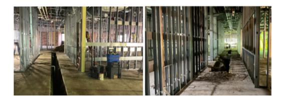
This week at Butler Junior High, we continued to frame the walls and soffits. The masons worked on the infills. Roofers have been working on replacing the gym roof. Electrical rough-in has continued. Underground plumbing for the kitchenette has been underway.
