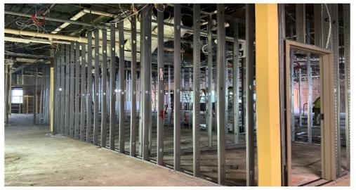
This week at Butler Junior High, we completed as much demolition as possible at this time. Framing has started in the library for the flex learning space. The masons have completed some masonry infills and will continue to work next week to complete their scope. Roofing materials were staged in preparation for the roofer's mobilization next week.
