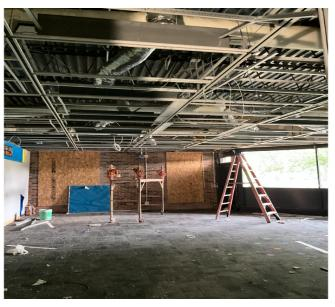
This week at Butler Junior High, we worked on demolition and underground plumbing exploratory. We completed demolition in the new kitchenette area in the District Office and will start saw cutting for the underground plumbing next week. Demolition at the Junior High included the removal of casework, select ceilings and select walls. Temporary lighting was also installed.
