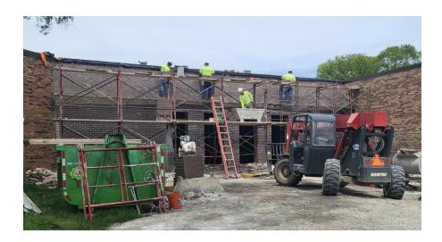
At Butler Junior High, the air & vapor barrier was applied to the CMU. The brick veneer was also completed. The masons have demobilized from the site, and we will work on condoning the construction area to a smaller footprint before graduation. We have gotten as far as possible with construction while school is in session. We look forward to having crews back on site once school is out for the summer. A site logistics plan has been established for the summer work.
